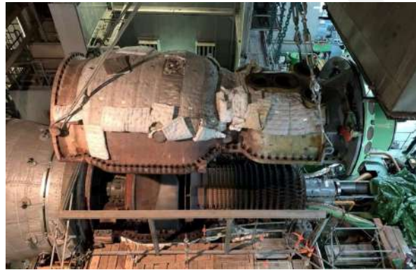
LIFTING OF GT CASING
